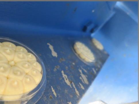
The upper flanges of the cross members were treated with 小島 *Bird Free* to prevent roosting (above left). As the pigeons especially favoured the corners of these flanges, the dishes were fixed closer together in each corner (above right).
