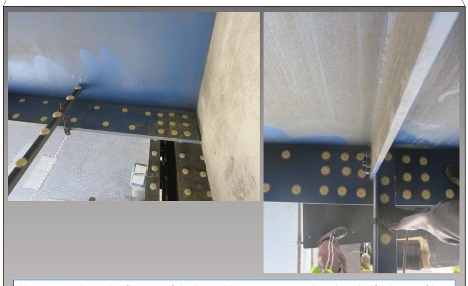
All corners where the flanges of the lateral beams meet the bearing shelf (above left), and the cross members (above right) were treated with nine dishes of 小島 Bird Free, as shown above, to prevent nesting.
