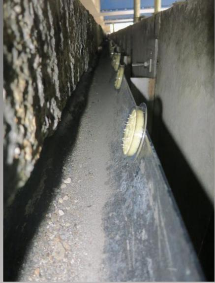
Both the ledge in front of the bearing shelf, and the gutter between that ledge and the bearing shelf were treated as shown above.
