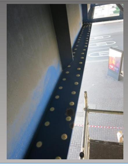
All 14 flanges between the bearing shelf and the pavement were treated with two rows of dishes of 小島 Bird Free, as shown above.
