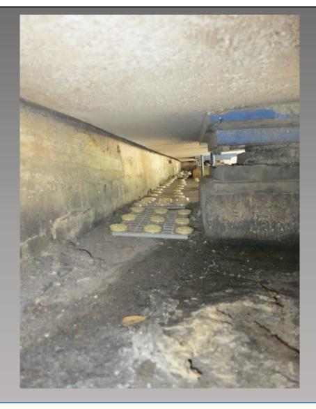
The corners of the bearing shelf, from which nests were removed, were treated with dishes of 小島  $Bird\ Free$  fixed to tiles (above left). To prevent pigeons from nesting behind the bearings, dishes of 小島  $Bird\ Free$  were applied as shown above right.
