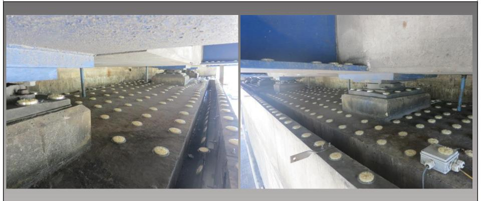
After removal of all faeces, the remainder of the bearing shelf was treated with dishes of 小島 Bird Free as shown above.
